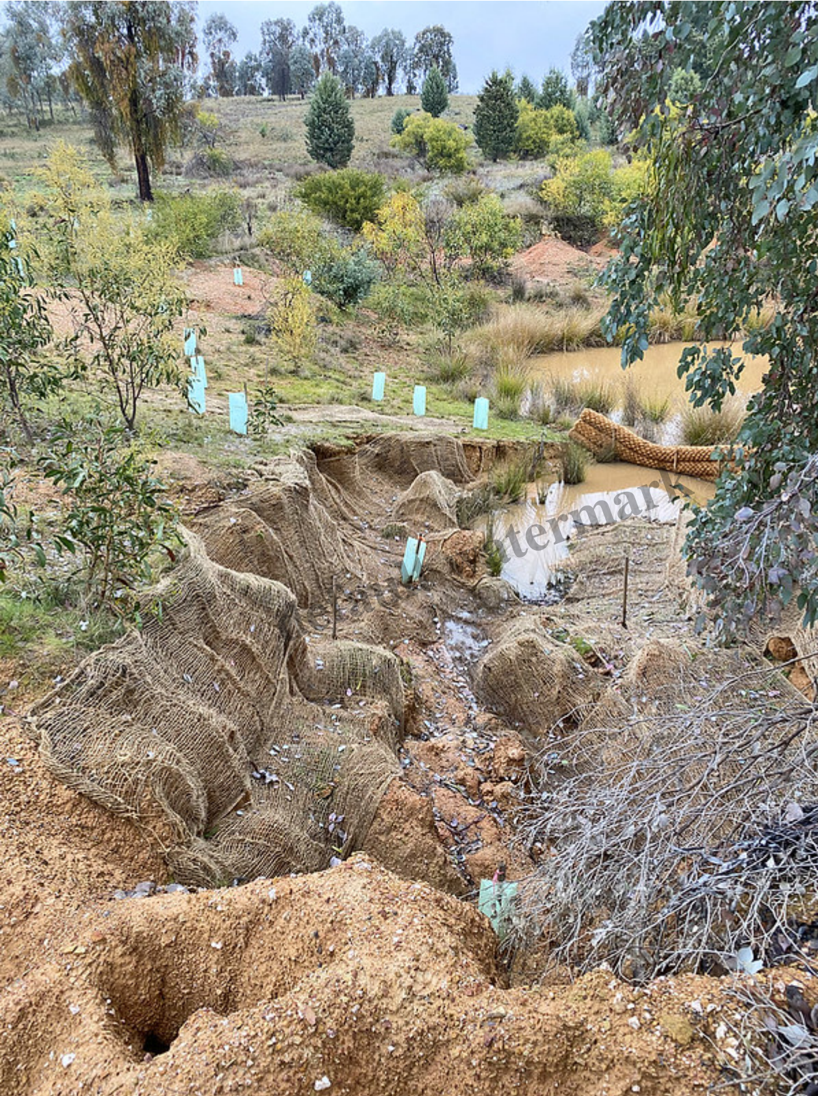
Matting has been installed to control erosion. Photos: Neville Bartlett
