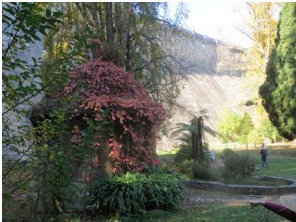
Dam wall from park, showing historic valve house
